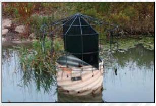
PERFORATED CSP RISER DROP INLET WITH ANTI VORTEX BAFFLE
